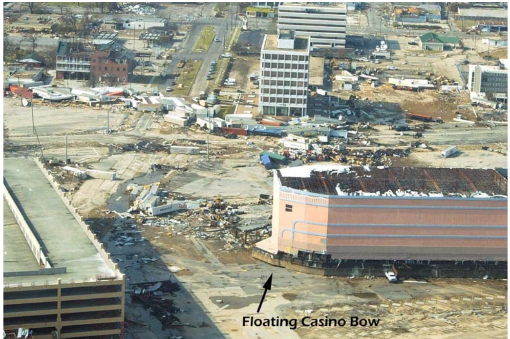
The big pink building is actually a displaced floating Casino, one of many destroyed in Gulfport, Mississippi during Katrina. It has floated on the storm surge a quarter mile from its original mooring. Photo USGS Hurricane Katrina Impact Studies, Post-Storm Quick Response Photos
