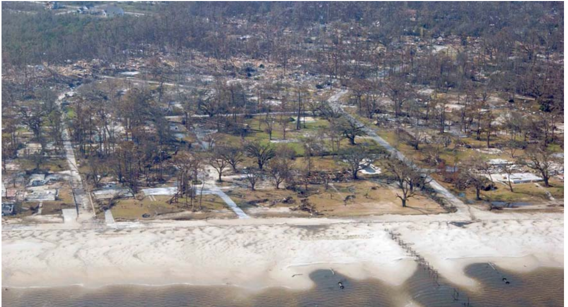
Gulfside, Beach Boulevard, Waveland Mississippi. Photo: USGS Hurricane Katrina Impact Studies, Post-Storm Quick Response Photos
