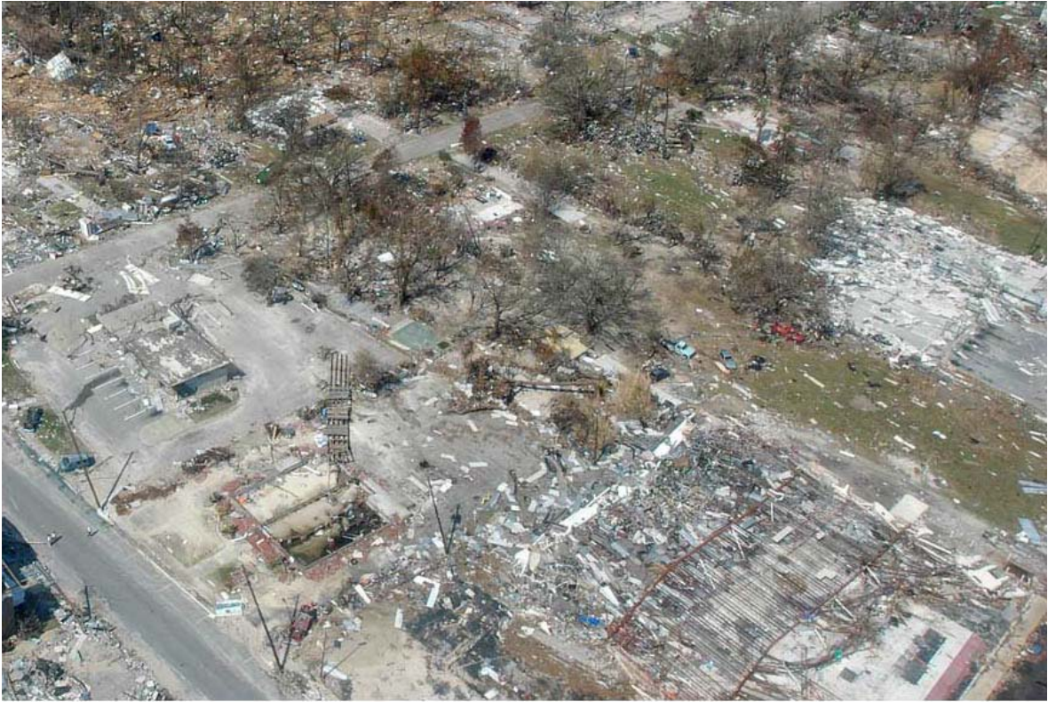
Gulfport, Mississippi, September 6, 2005: Damage from Hurricane Katrina. Photo Credit: Federal Emergency Management Administration
