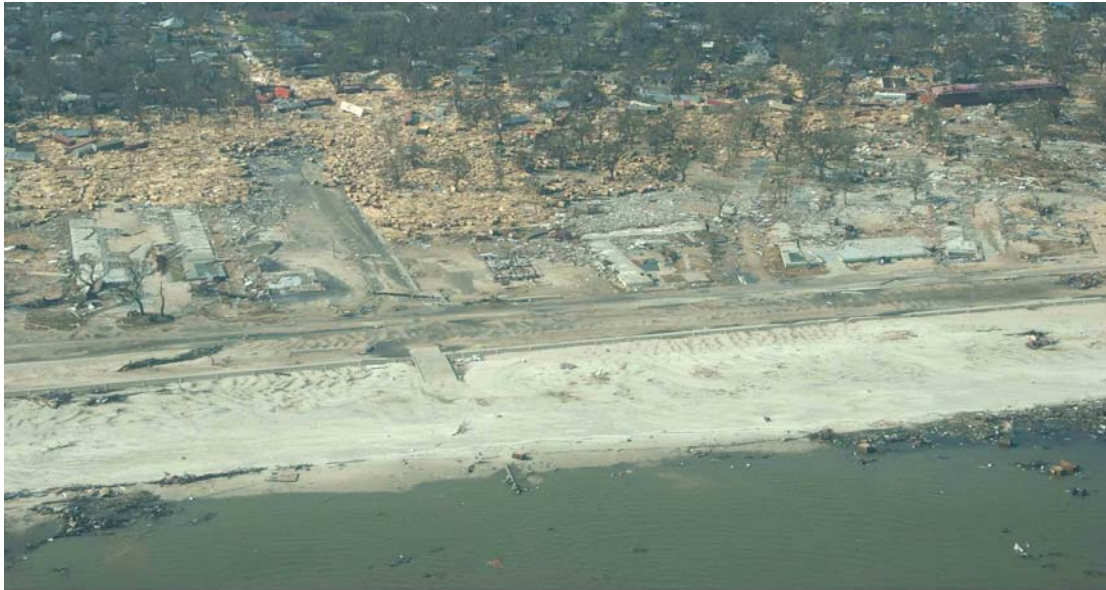
Broad Avenue at Beach Boulevard, Long Beach, Mississippi (Gulfport). Photo: USGS Hurricane Katrina Impact Studies, Post-Storm Quick Response Photos
