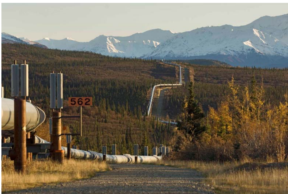
The Alaska Pipeline
